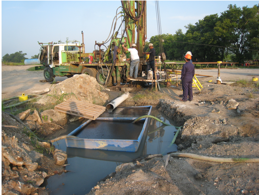
Simple Gravity Segregation Mud System
