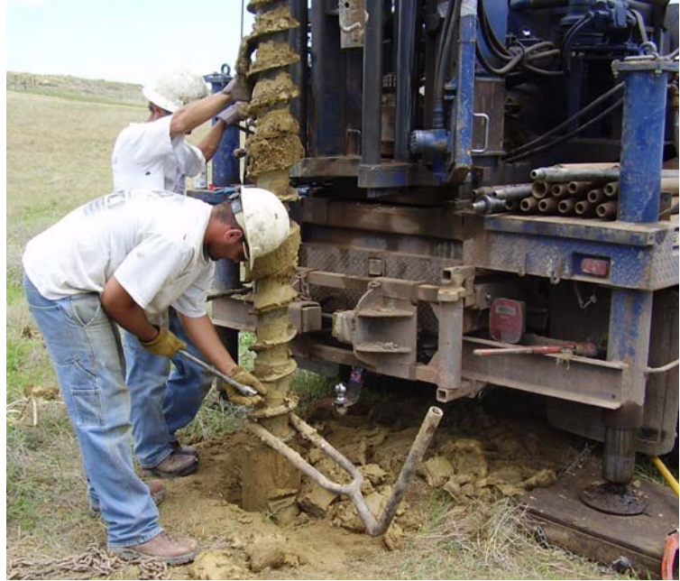
Hollow Stem Auger Boreholes in the Prairie Dog Creek Watershed, Wyoming
