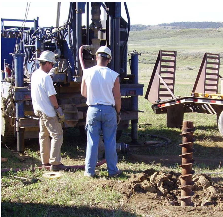
Monitoring Well Drilling Prairie Dog Creek Watershed, Wyoming
