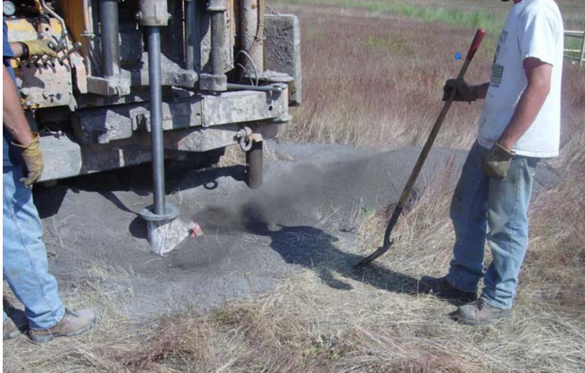
Air Rotary Drilling LX Bar Creek Watershed, Wyoming
