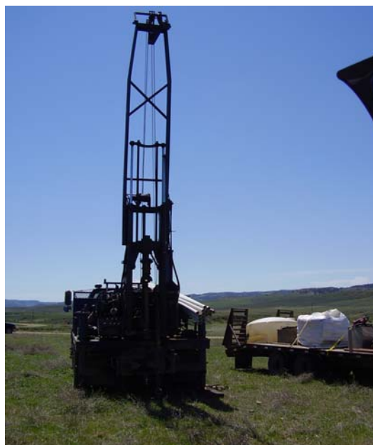
Water Well Drilling Rig Used To Install Monitoring Wells PRB, WY
