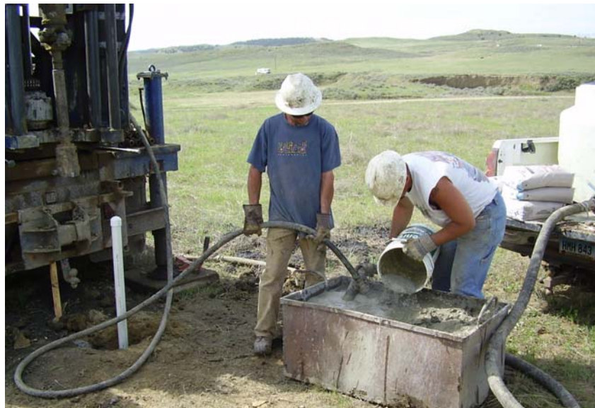
Grouting Monitoring Wells in the Prairie Dog Creek Watershed, Wyoming
