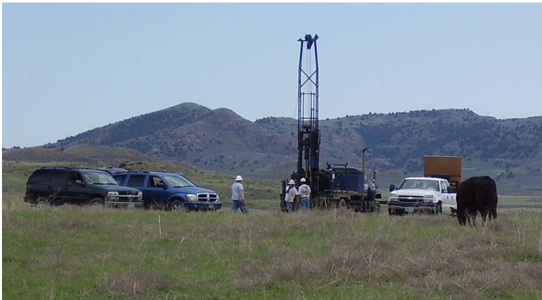
Drilling below an On-Channel CBNG Impoundment in the Prairie Dog Creek Watershed, Wyoming
