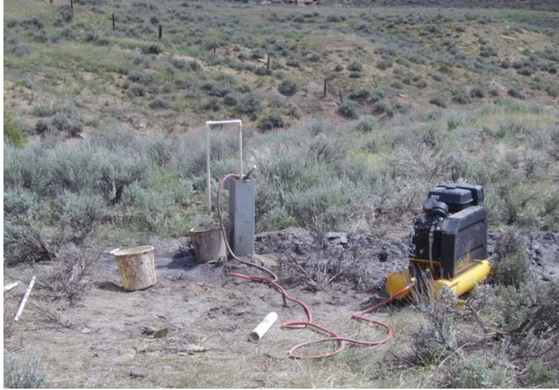
Monitoring Well Development in the Prairie Dog Creek Watershed, Wyoming
