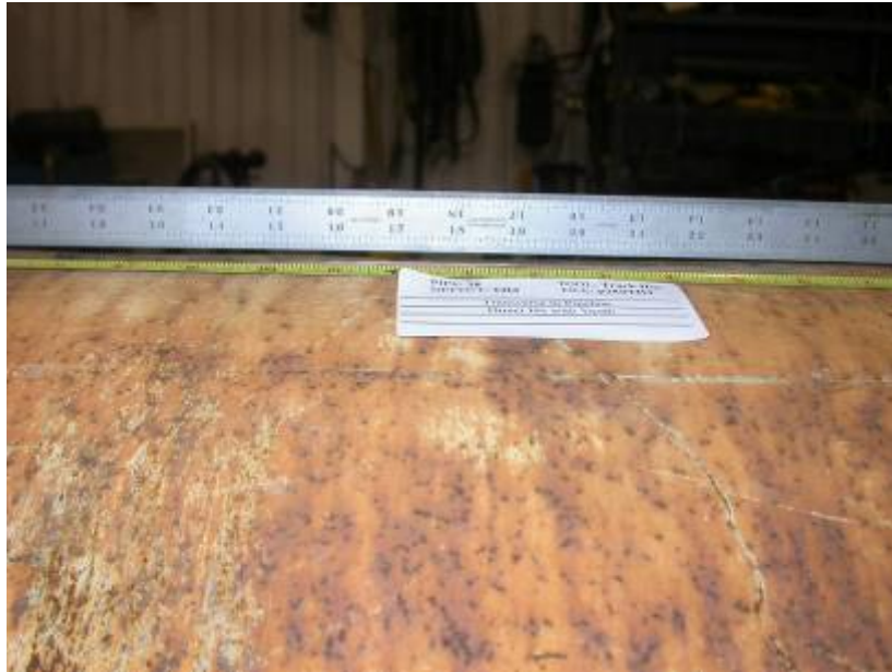
Figure 3-15. Defects D7, D8, D9 (p28dTH4)
