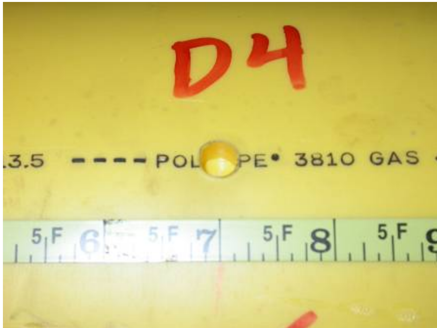
Figure 5-6. Defect D7 (D4)
