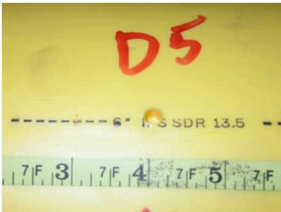
Figure 5-7. Defect D10 (D5)
