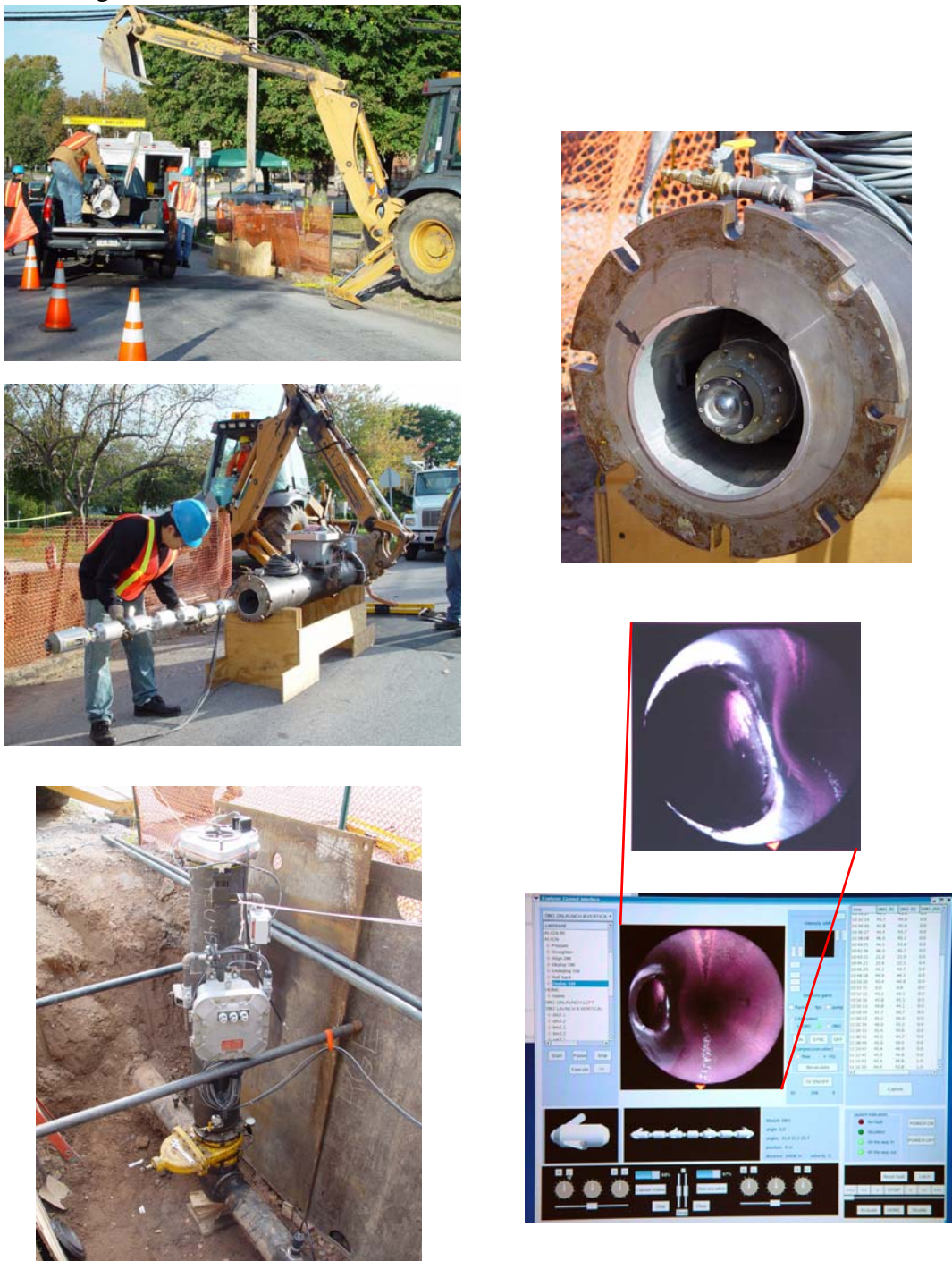
Figure 34: Live high-pressure steel main deployment images
