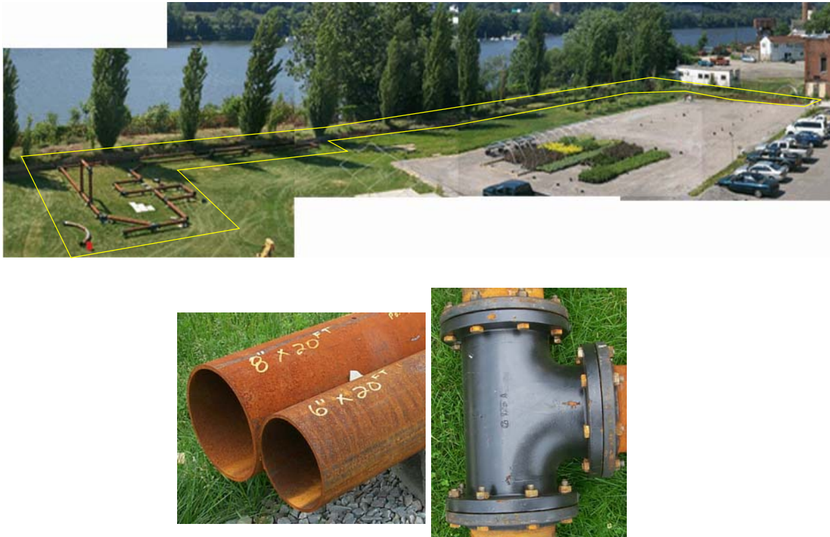
Figure 29 : View of the test pipe-network setup at CMU (inside yellow box)
