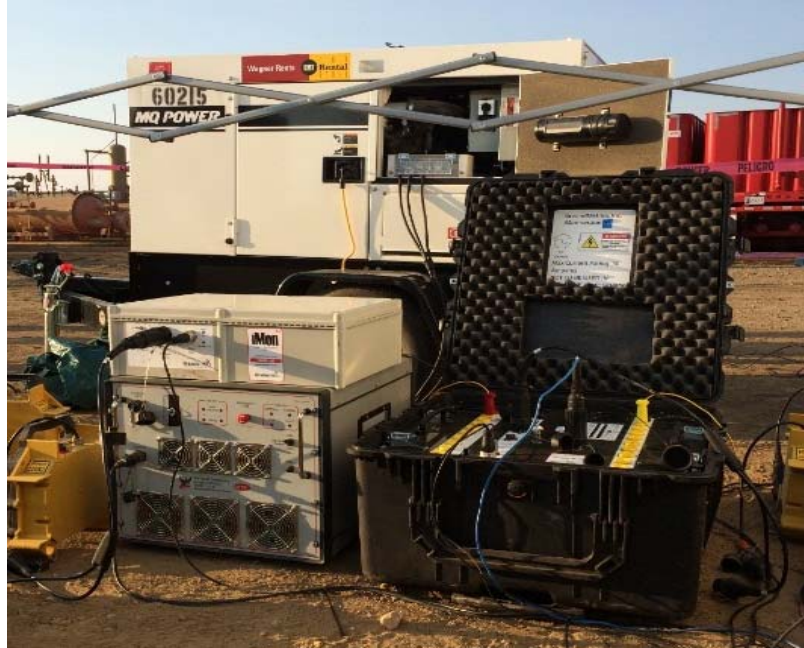
Figure 19. The DSR source transmitter (front left), two channel current monitoring unit (front right) and electrical generator (rear) as deployed at the site during the fracturing experiment
