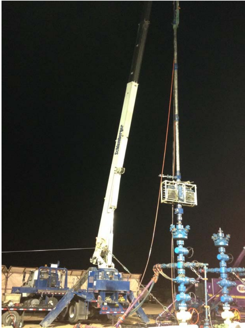
Figure 20. Downhole electrode installation into the well
