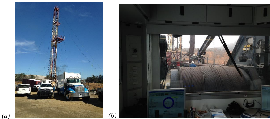
Figure 2. (a) Workover rig for installing 7.30 cm (2.875 inch) tubing in well. (b) Wireline for lowering and raising downhole camera, sidewall coring device, and the isolation behind casing scanning tool (IBC).
