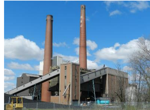
90 MW T.B. Simon Power Plant
