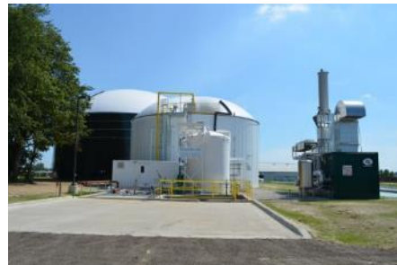
CSTR system (2000 m 3 , 0.5 MW)
