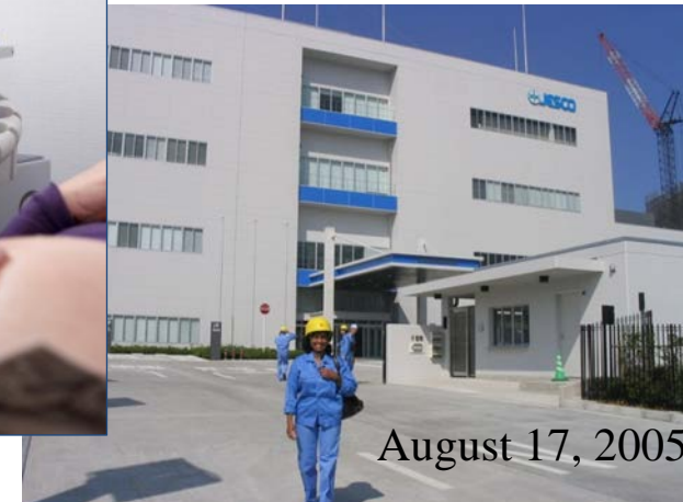
AHO Facility for waste water treatment plant at The Tokyo Bay, operated by JESCO
