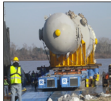
Confidential Client Ammonia Plant Expansion Donaldsonville, LA
