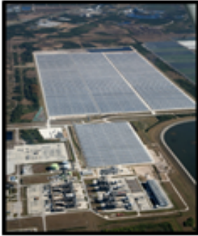
Florida Power & Light Hybrid Solar Power Facility Indiantown, FL
