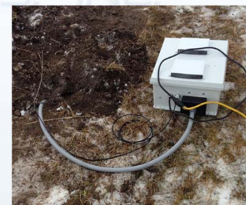
Near-surface leaks into the atmosphere
