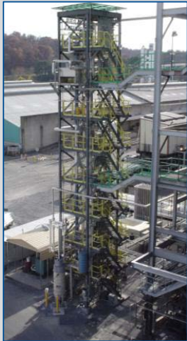
RTI PILOT PLANT TEST UNITS AT EASTMAN COAL GASIFICATION PLANT
