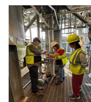
Installation of Amine Degradation Sensors onto SSTU in March 2024
