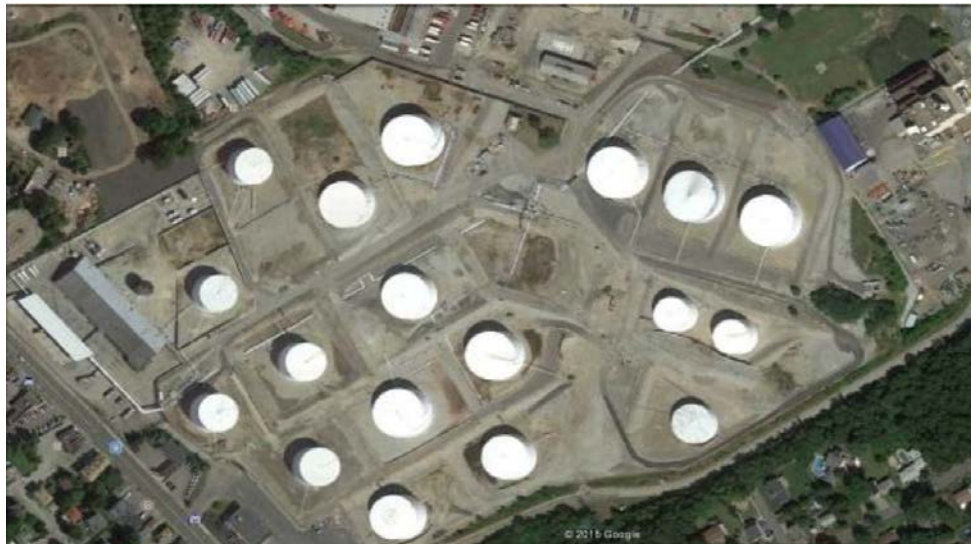
Exhibit 4-16 Overhead View of Plant 3 (15)
