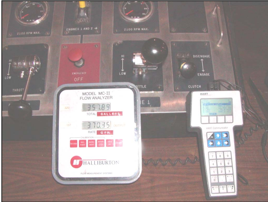
Figure 20. Flow control console, flow meter, and pressure readout
