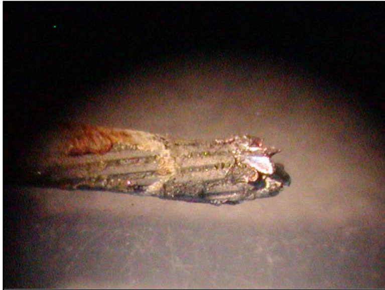
Figure 27. Example of poor soldering quality for wire connections
