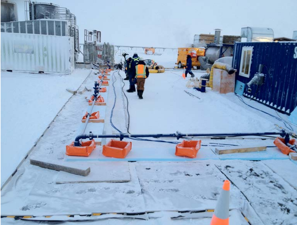
Figure 24: Construction of high-pressure hard line on blue-board insulation base
