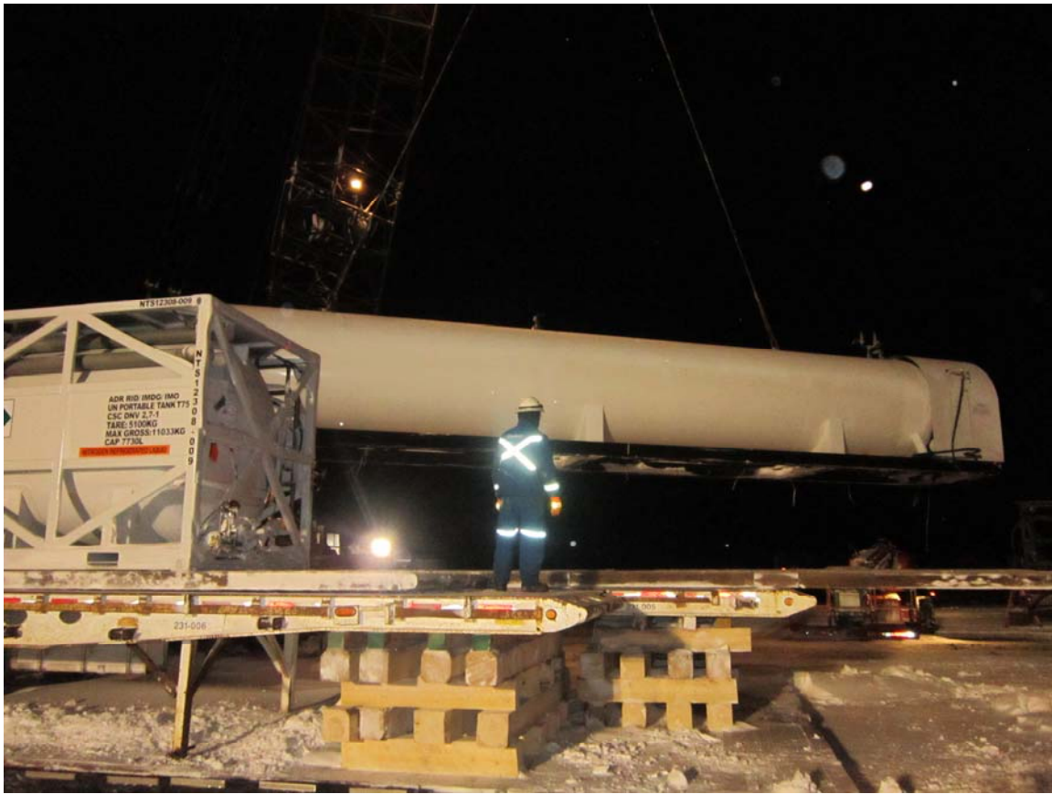
Figure 22: Spotting carbon dioxide tank at Igñik Sikumi #1
