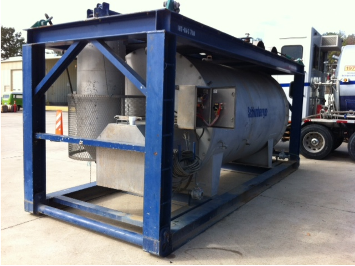
Figure 23: Diesel-fired Glycol/Water Heater
