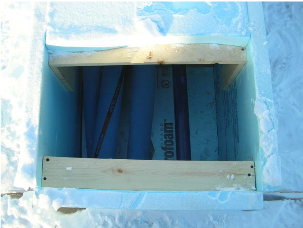
Figure 25: View inside blue-board insulation tunnel
