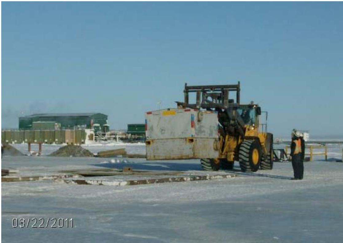
Figure 4: Cellar-setting operation; PBU L-pad facilities in background
