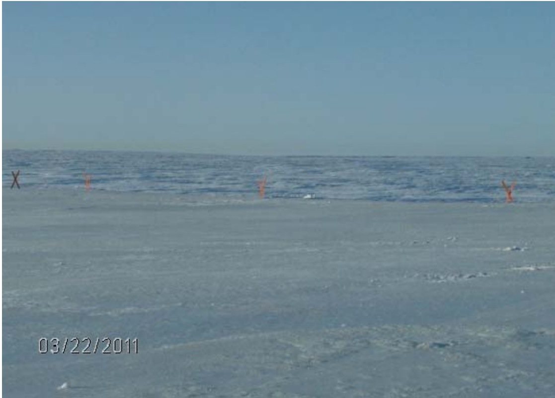
Figure 3: Ice-pad construction completion
