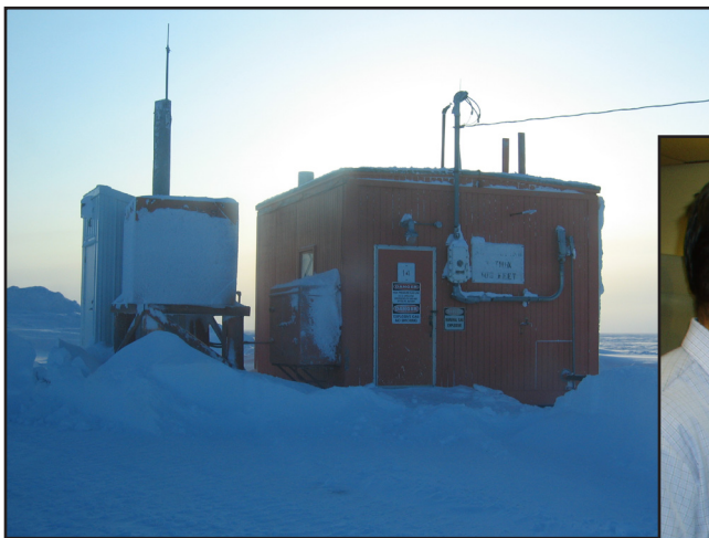
Figure 3. Well housing and methanol tank (methanol injection is used to mitigate hydrate formation in the production string) at the East Barrow No. 14 well.
