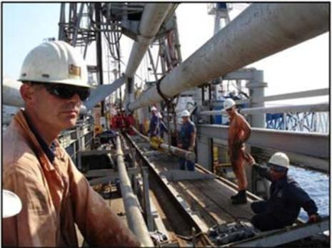
Assembly of the FPC takes place on deck of the drill ship in a horizontal position
