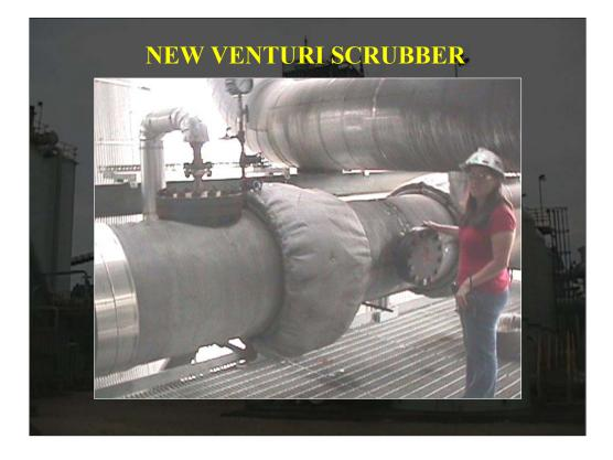
We have also installed an additional venturi scrubber upstream of the COS hydrolysis KO drum. This provides protection for the COS hydrolysis superheater and catalyst bed from particulate fouling in case the upstream syngas scrubbers malfunction.
