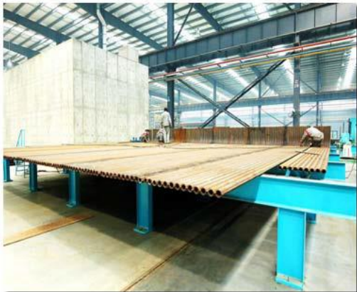
Straight flat panels in shop.
