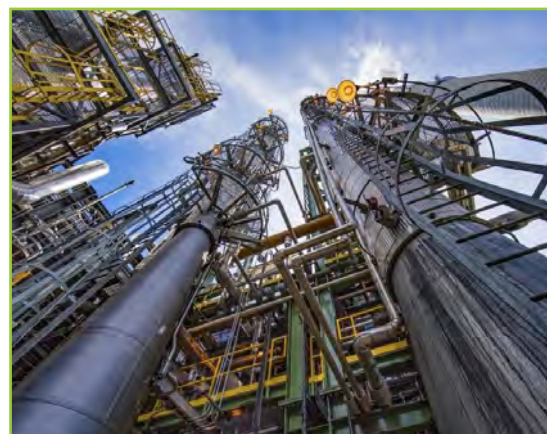
Petra Nova in Texas (USA) is the world's largest post-combustion carbon capture system, capturing CO 2 produced by burning coal for use in enhanced oil recovery (EOR).
