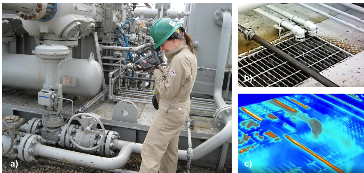
Figure 2-5. a) Screening a pneumatic device with the FLIR OGI Camera, b) compressor rod packing vent, c) FLIR view of compressor rod packing vent
