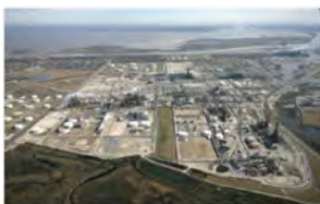
Port Arthur 1 & 2 Hydrogen Production Plants
