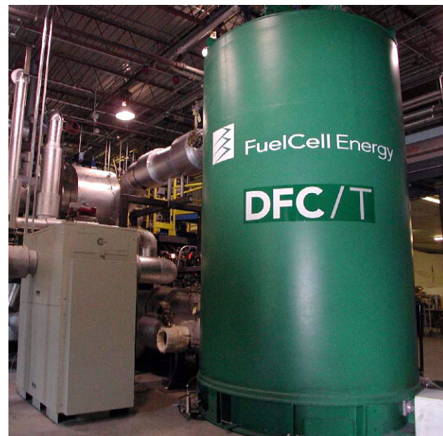
Figure 1. Sub-MW DFC/T Hybrid Power Plant Showing Full-Size DFC Stack Integrated with a Capstone Micro-turbine
