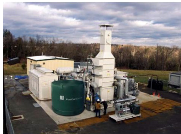
Figure 1. MW-Class Module Performance Testing at Torrington Facility (Operation at rated load, on natural gas, verified.)
