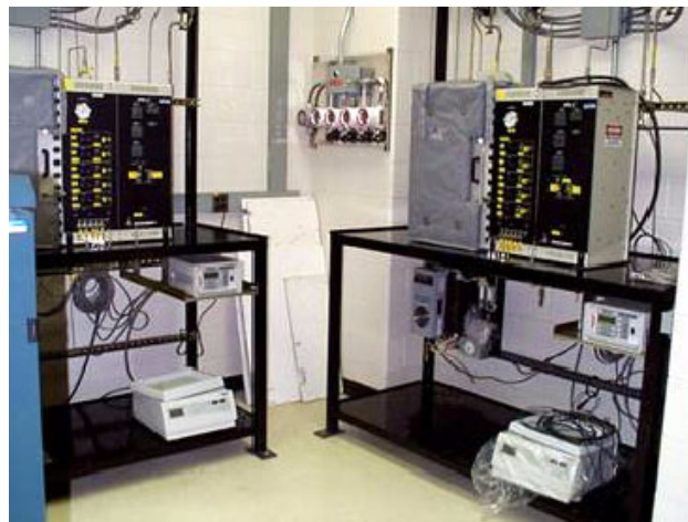
Figure 1. Catalyst Test Facility
