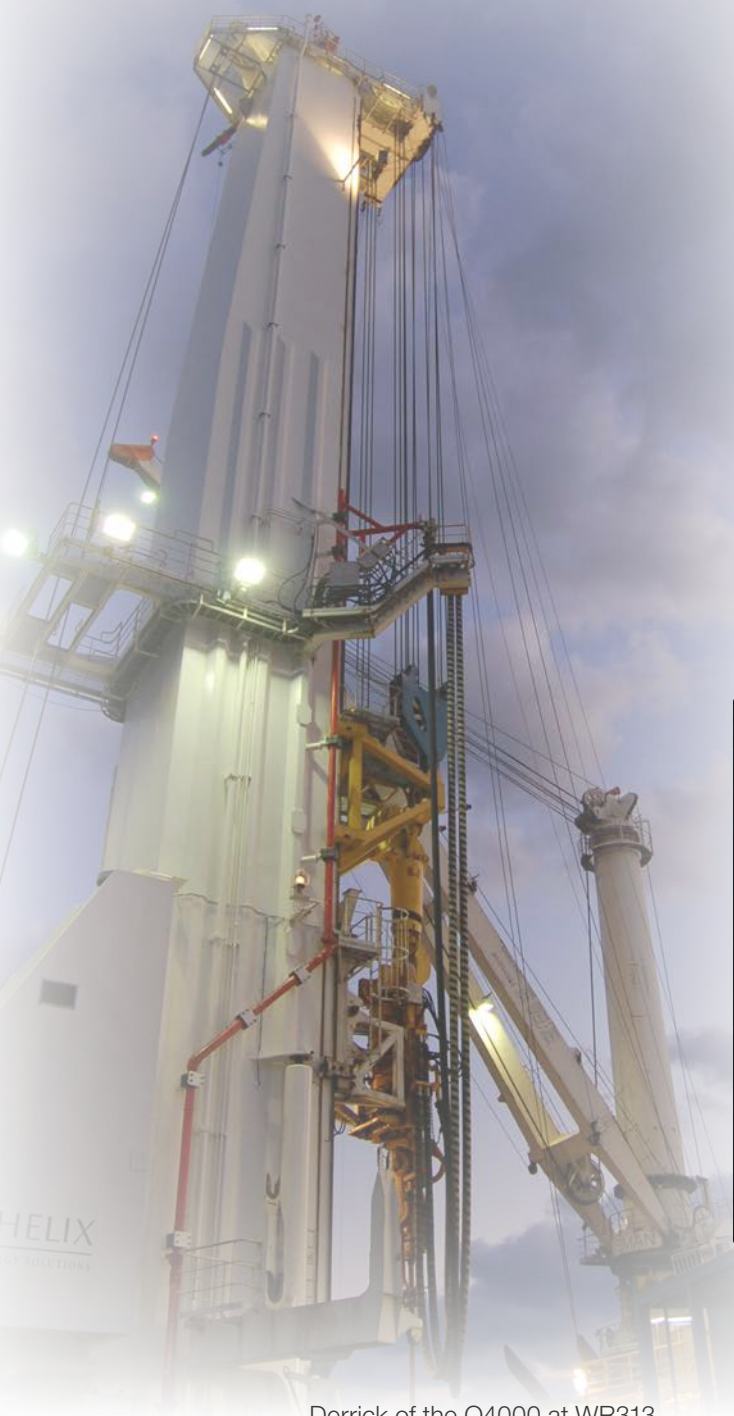
Derrick of the Q4000 at WR313.
