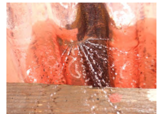
Cracks in transversal direction
