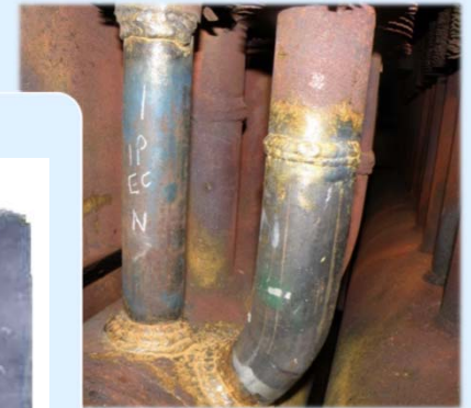
Oxidation/Corrosion
