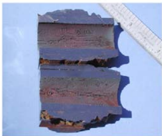
Waterwall web cracking
