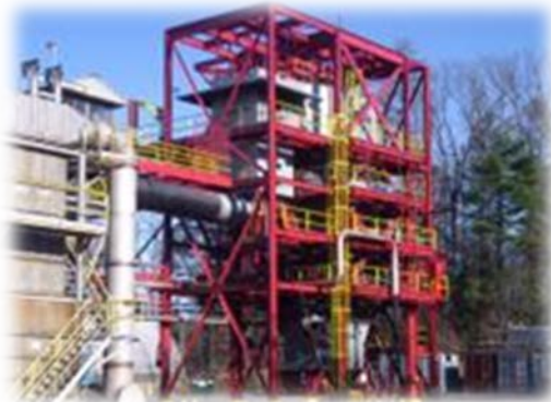
5 MWE Oxycombustion Pilot
