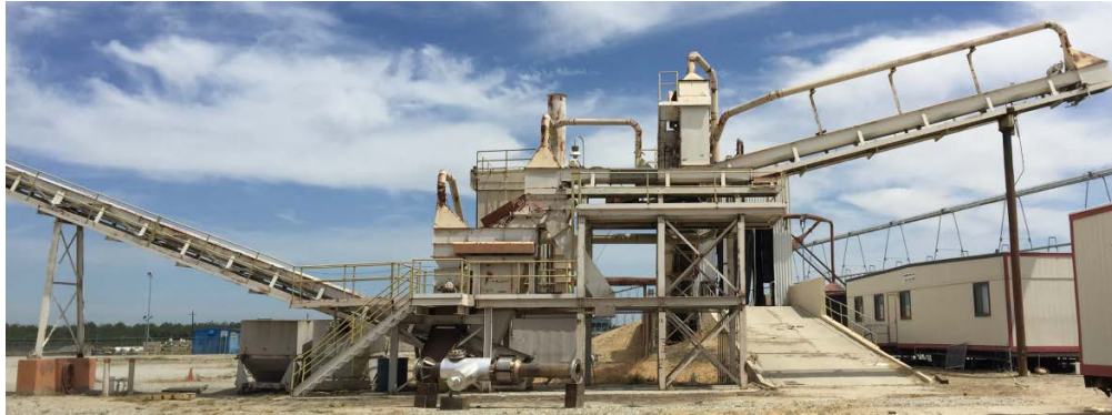
Existing biomass unloading station, conveyors, and storage silos
