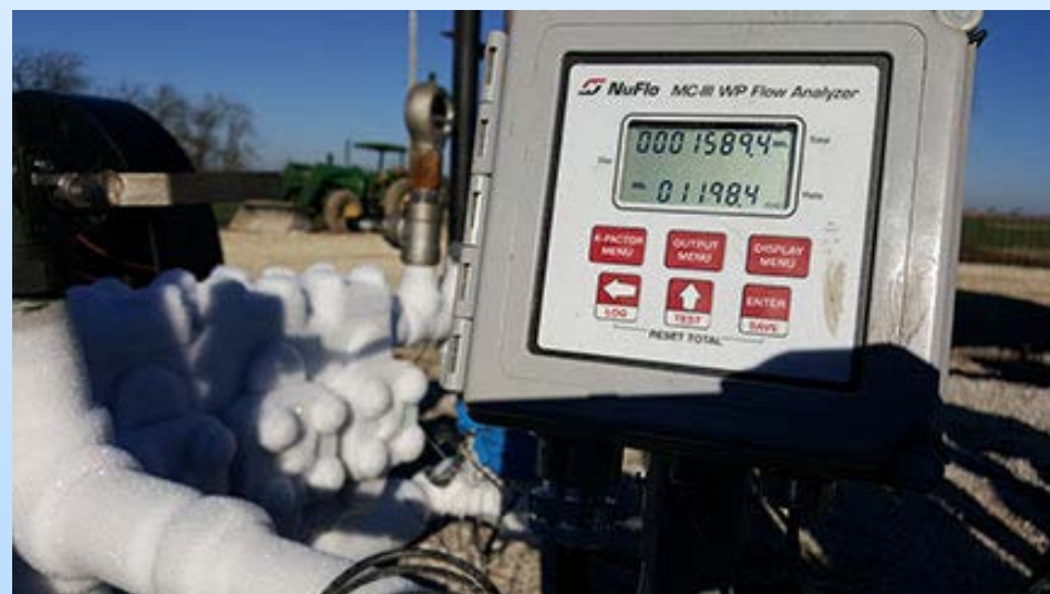
SCADA System installed on wells
