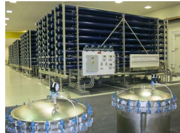
RO production train, North Cape Coral RO Plant
