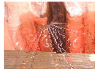
Cracks in transversal direction
