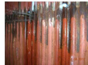
Cracks in longitudinal direction
