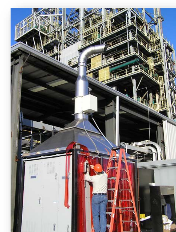
PILOT PROJECT FUEL CELLS
