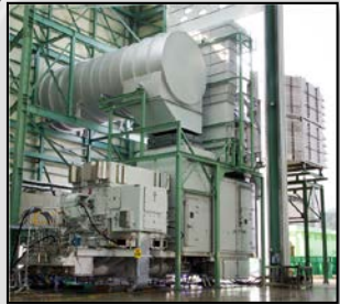
Gas Turbine & Compressor Packages
