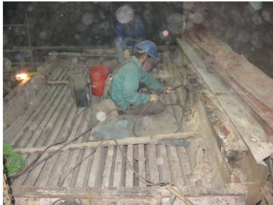
INSTALLATION OF ENVIRONETIX SENSORS IN MERC POWER PLANT
