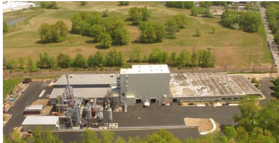
Aerial View of Alstom R&D Test Facilities May 2015
