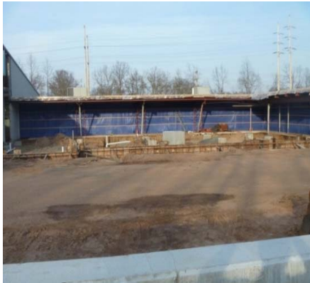
Cut Opening - April 2014
