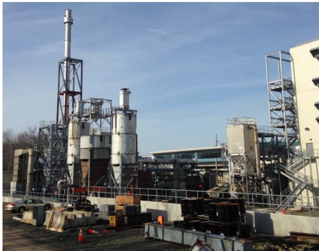
Outside Equipment Complete March 2015
