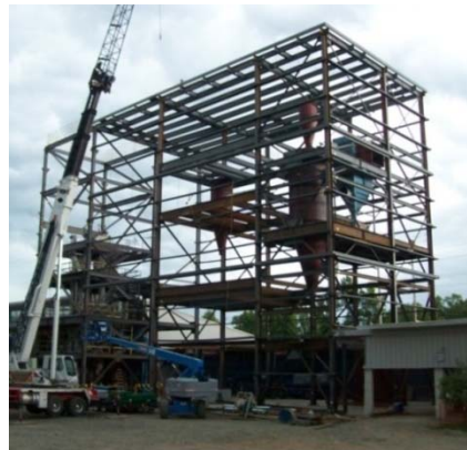
Tower Steel - June 2014
