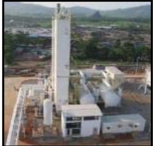
Air Separation Unit
