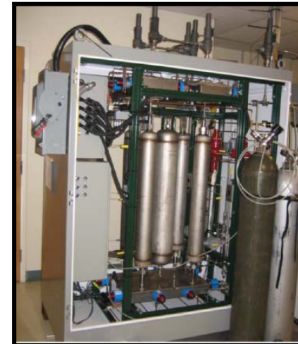
TDA Shift/Separation Skid
