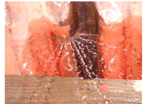
Cracks in transversal direction
