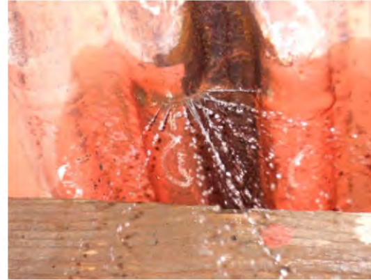
Cracks in transversal direction
