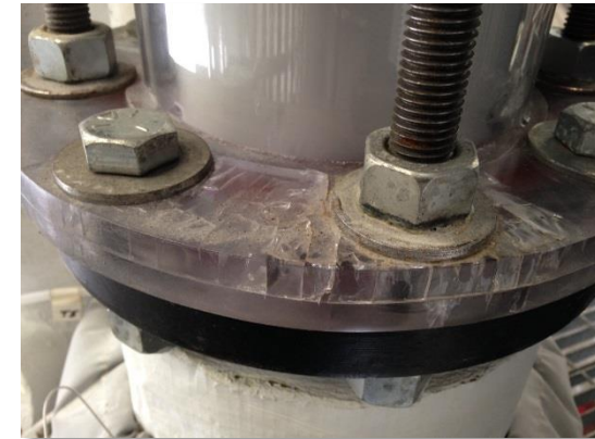
Mechanical failure of PC viewp
