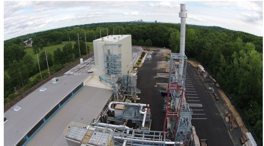
Aerial View of Alstom R&D Test Facilities June 2015
