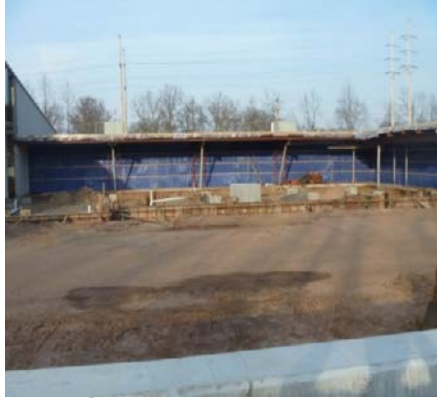
Cut Opening - April 2014
