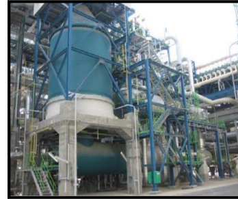
Secondary AutoThermal Reformer
