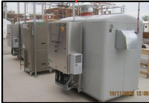
PX Syngas Generators (simulate coal syngas)
