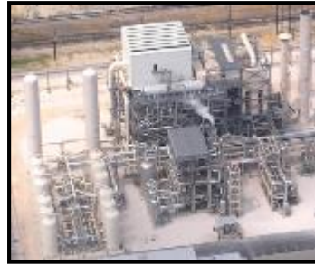
Primary Steam Methane Reformer
