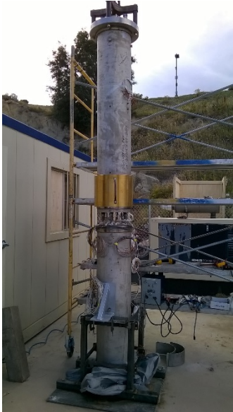
30 ft of HEX + stack modules assembled and installed down hole
