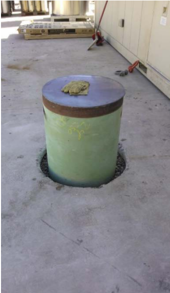
32 ft liner installed
