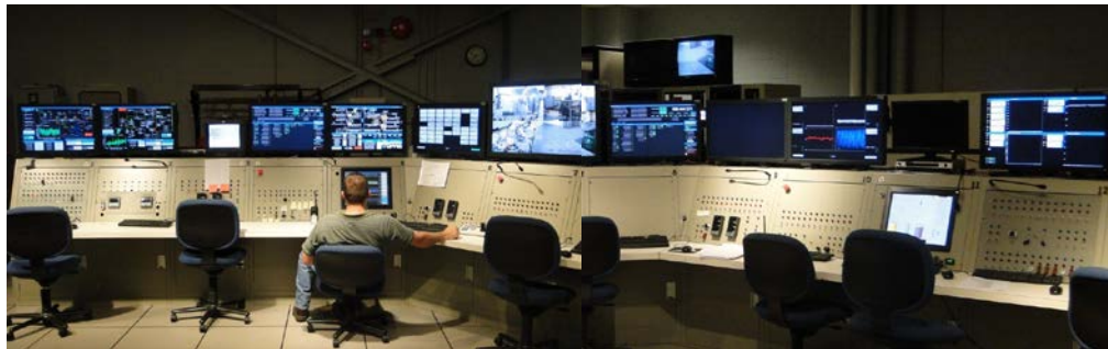
Remote operation from central control room
