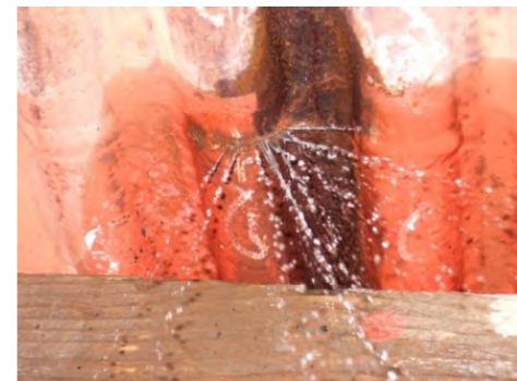
Cracks in transversal direction
