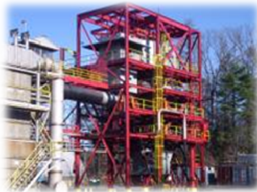
5 MWE Oxycombustion Pilot
