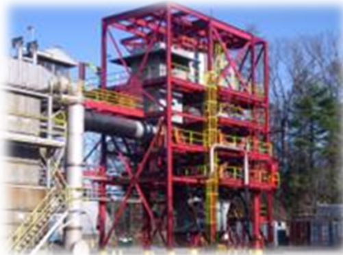
5 MWE Oxycombustion Pilot
