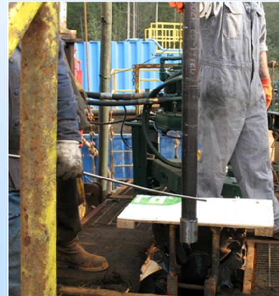
Top: Flat pack containing fiber optic cable. Bottom: Terminus of the fiber optic cable as it is being deployed in the well
