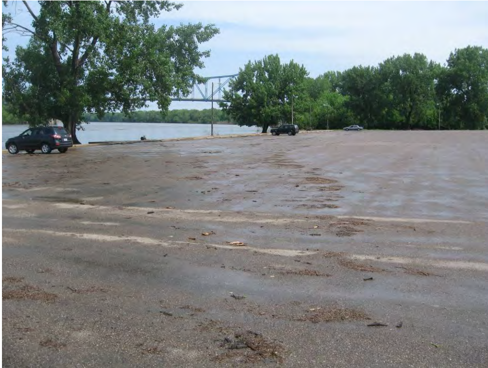
Photo 1. Drift Line Observed in parking lot at Village Property (Area 1).
