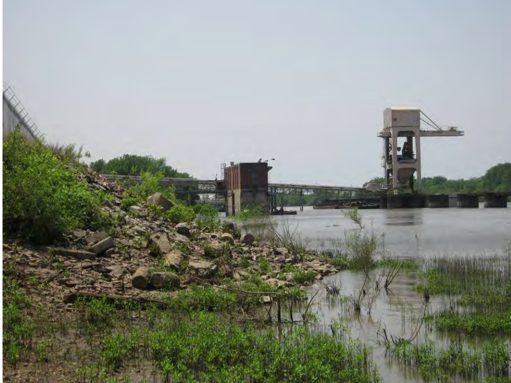
Photo 7. Looking downstream from Area 3 at existing coal unloading operations.
