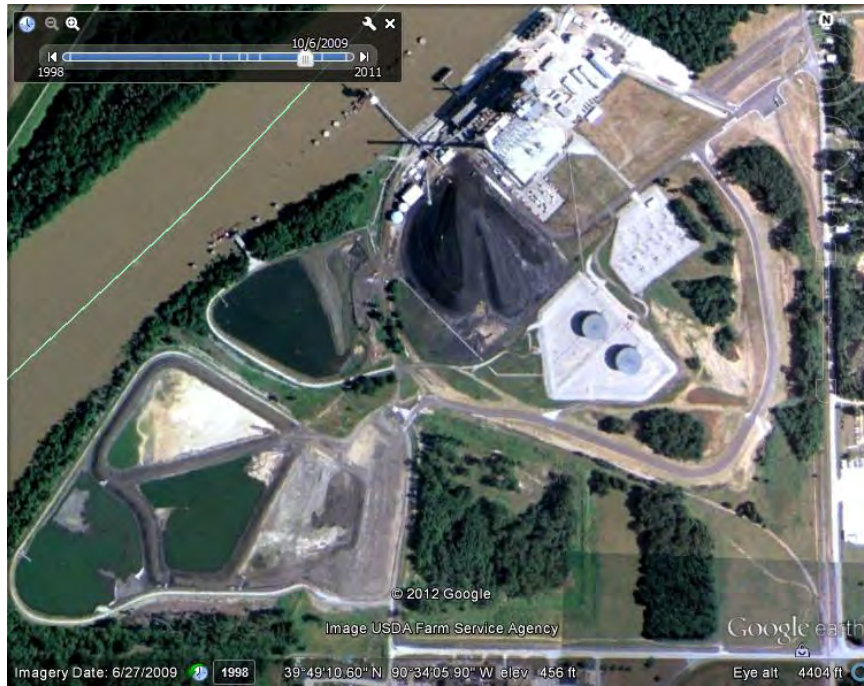
Photo #2 Meredosia Energy Center 2009 Google Earth 2012
