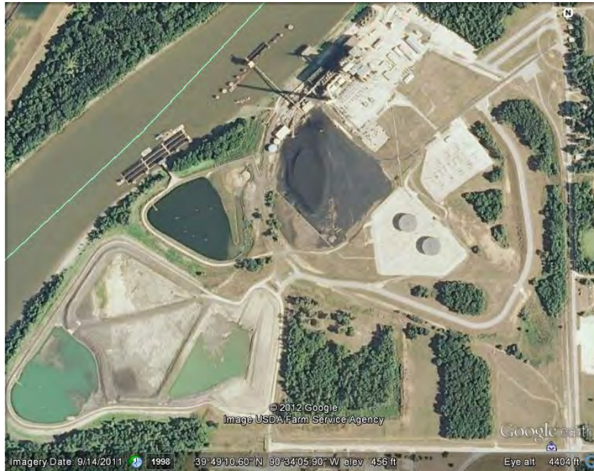
Photo #1 Meredosia Energy Center 2011 Google Earth 2012
