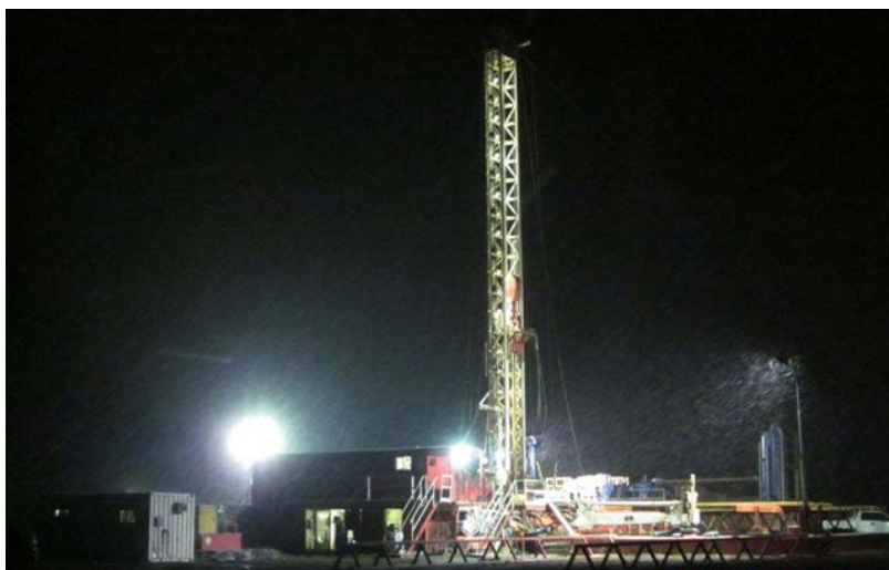
Figure 2-28. Drill Rig during Nighttime Operations
