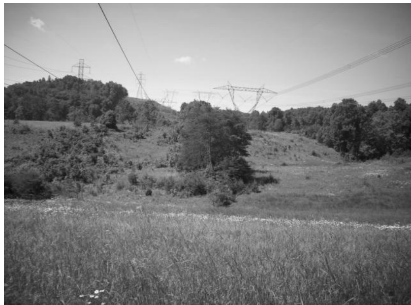
Figure 3.8-3. Previously Disturbed Vegetation Community Occupying Existing ROW along the South Pipeline Corridor – Segment D
